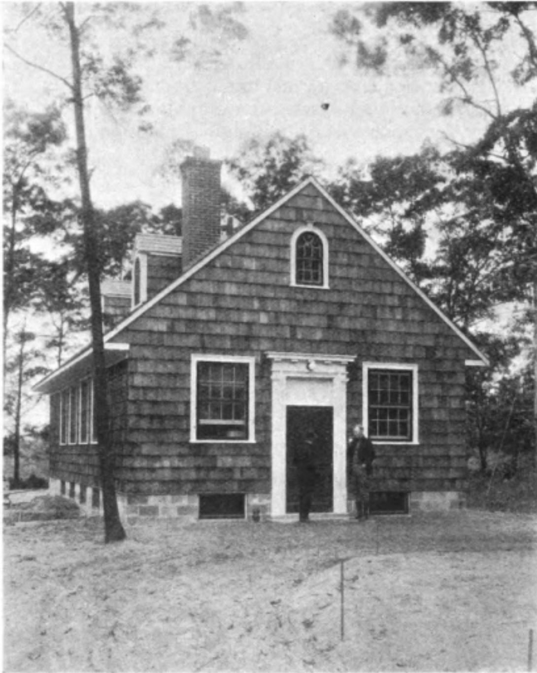
FIG. 2.—Exterior View of Receiving Station at Riverhead, L.I.
